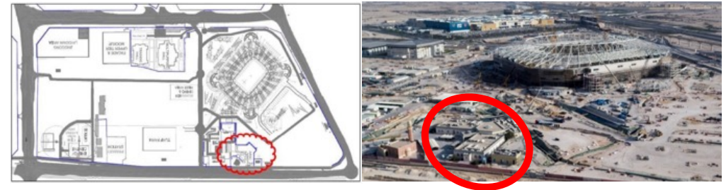
Figure 11: Ahmad Bin Ali Stadium's usage of existing buildings
