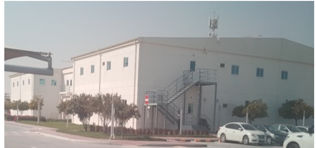
Figure 10: Lusail Stadiums' site office
