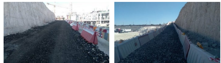
Figure 11 : Hauling roads paved with milled asphalt
