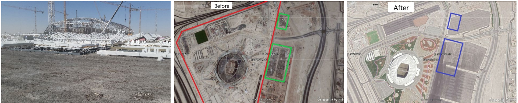
Figure 5: Application of prime coat on laydown area at Al Janoub Stadium
