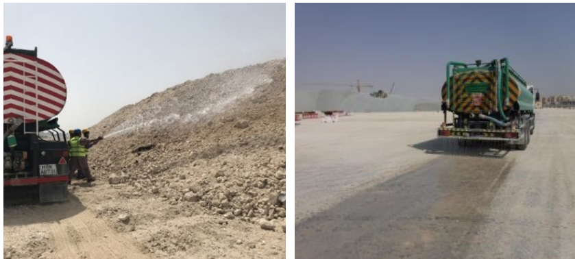
Figure 14 : Water spraying for dust suppression
