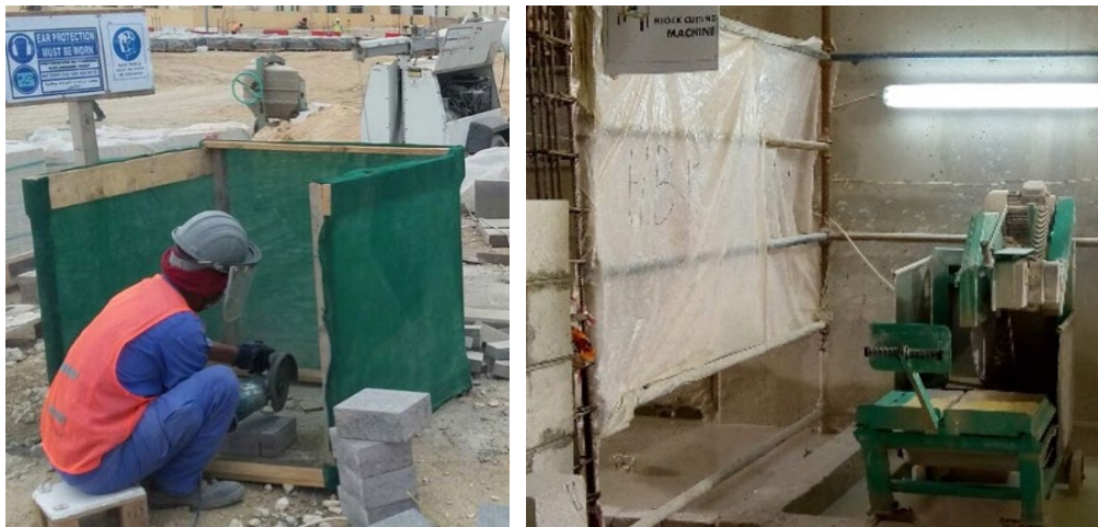
Figure 25: Barriers around dust-generating equipment
