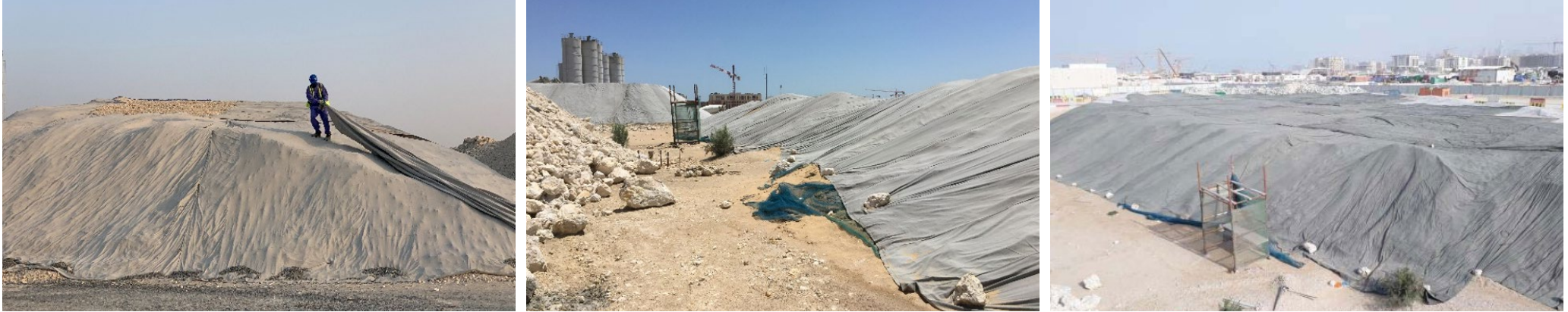
Figure 9 : Long-term stockpiles covered with tarpaulin
