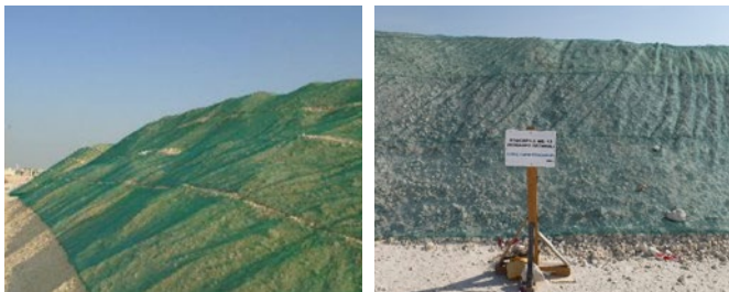
Figure 20 : Covered stockpiles with plastic net
