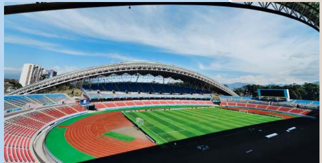
National Stadium of Costa Rica: San José
