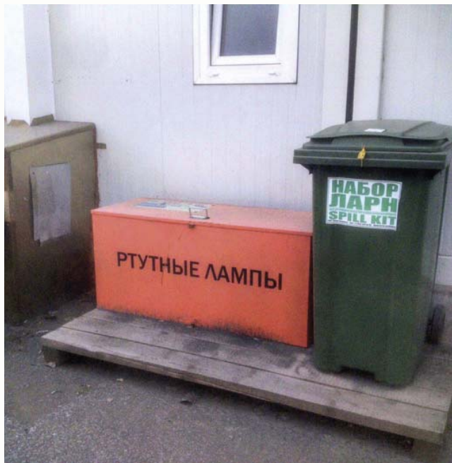
Used luminescent and mercury lamps are collected in a dedicated airtight container, and further protection of the broken lamps is provided by means of separate sealed tubes to prevent contamination by mercury fumes.
