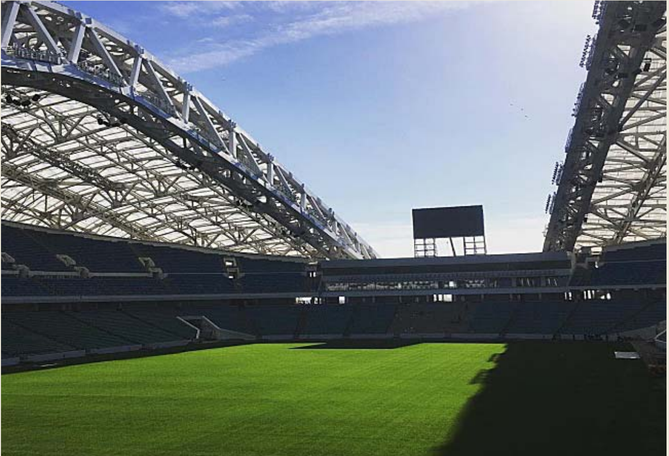
Innovative translucent membrane of ETFE material
